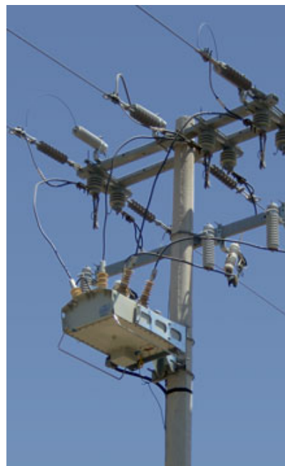
An Automated Circuit Recloser
